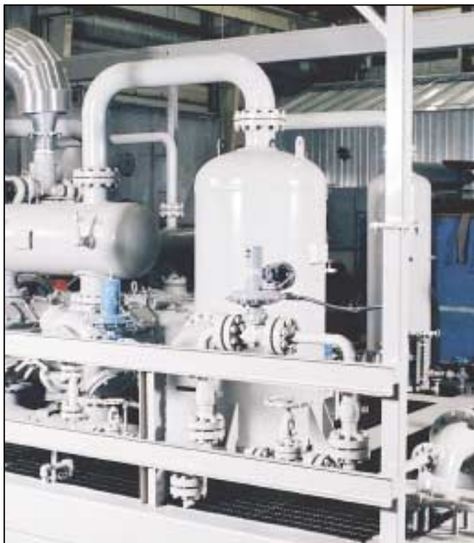
Figure 1. Typical vertical knockout drum
